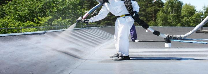
Silicone Seal 3000 Roof Coating is the second membrane Superior Seamless Roofing applies. It is a high solid non VOC liquid silicone that is the UV protection for our Expandothane membrane. It also acts as a secondary waterproofing system. Silicone Seal 3000 is a highly reflective roof coating that does not absorb solar radiation the way traditional roofing systems do.
